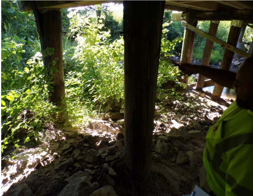
BENT # 3 PILE "C" SPLIT
