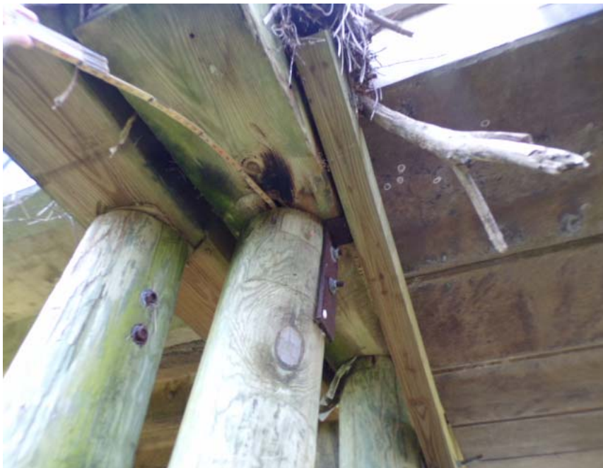
BENT # 1 "B" CAP DECAYED
