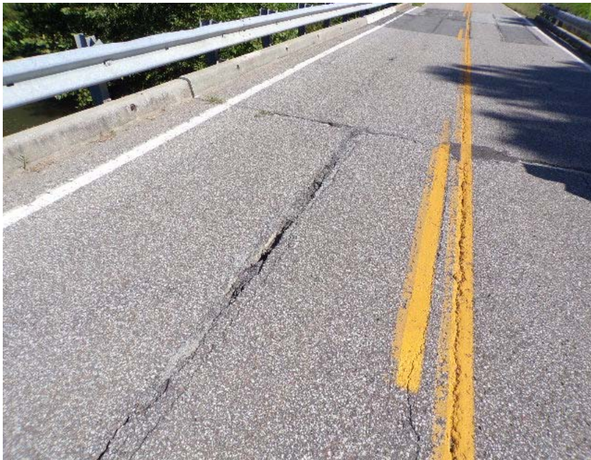
SPAN # 1 SETTLING
